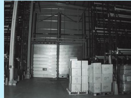
Warehouse with IR Illumination
